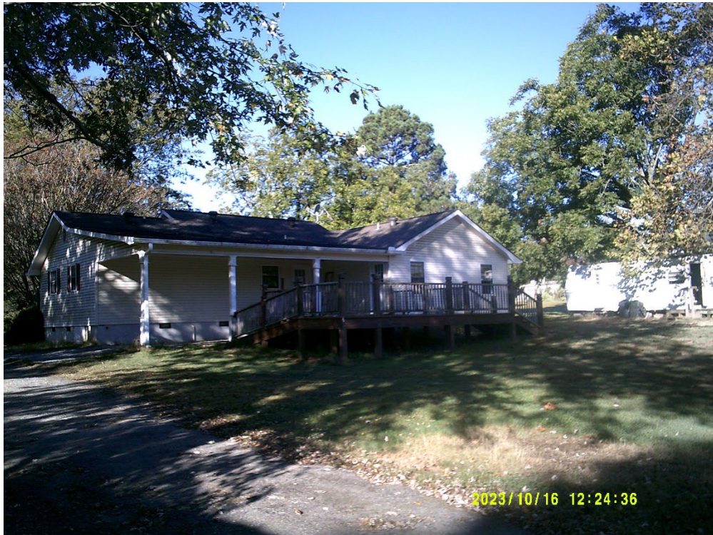
Rear View of Existing Primary Dwelling
