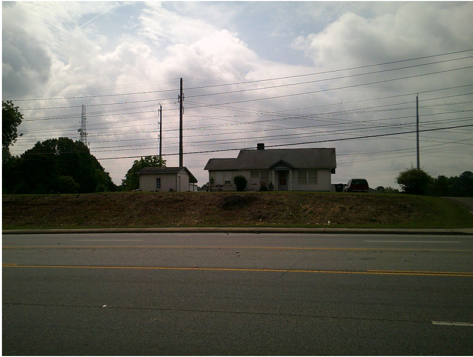
View of the Site from Buford Highway
