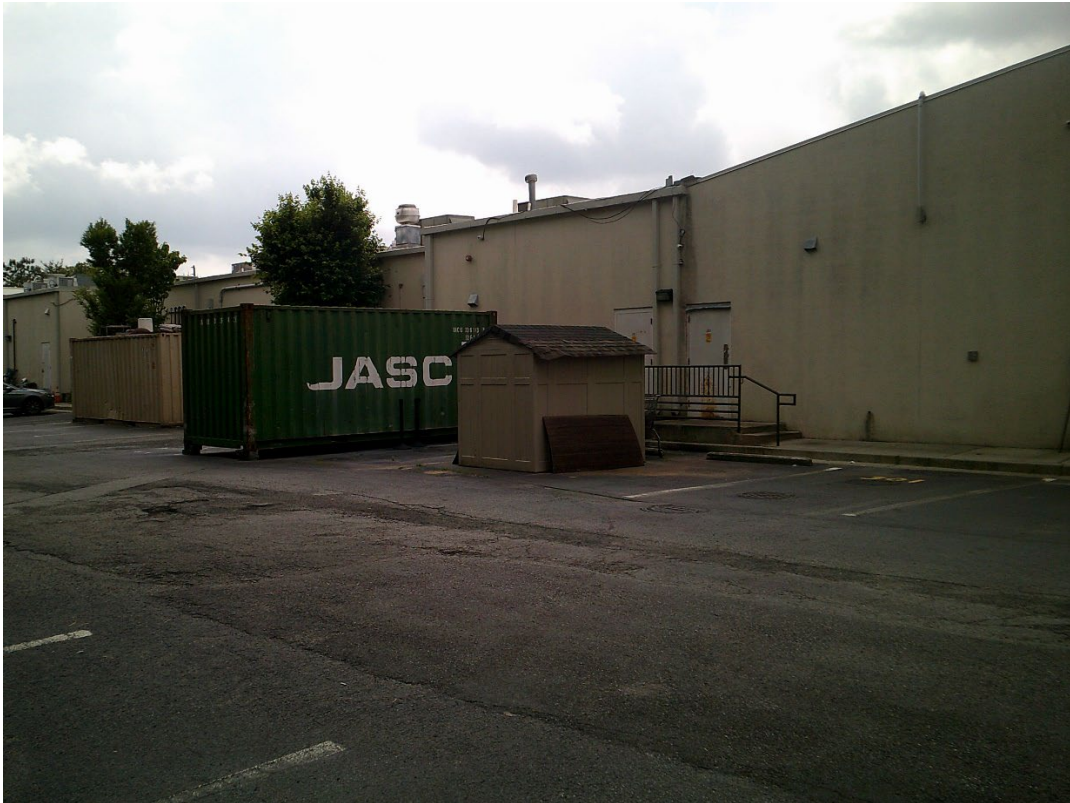
View of Storage Containers Located in the Rear
