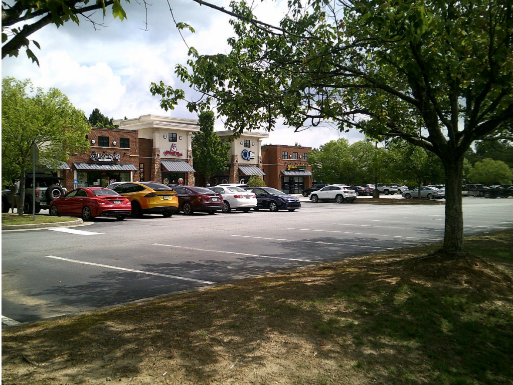
View of Existing Retail Business off Old Norcross Road
