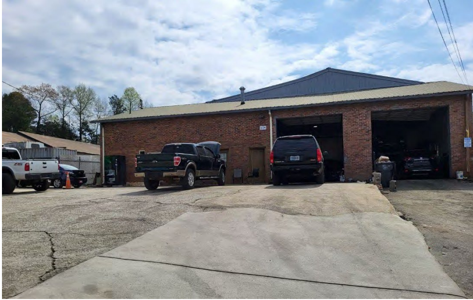
View of the existing building
