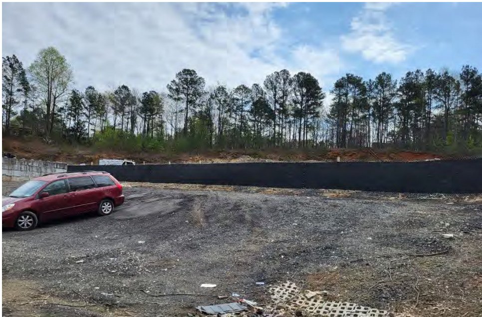
View of fence under construction
