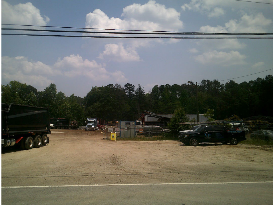
View of Site Entrance
