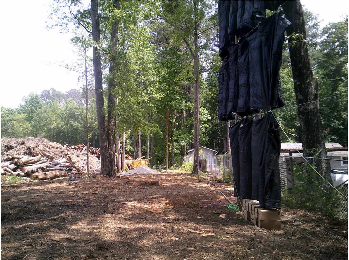
View of Screening System Used by the Site
