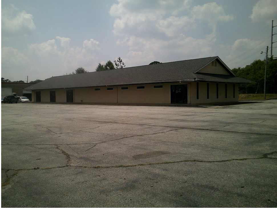
View of the Existing Office Building
