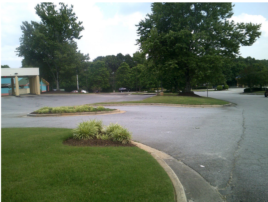
View of Existing Site Entrance
