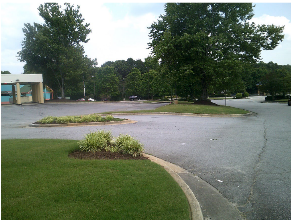
View of Existing Site Entrance
