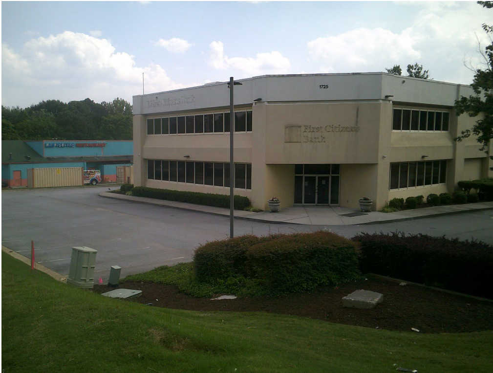
View of Existing Building from Indian Trail
