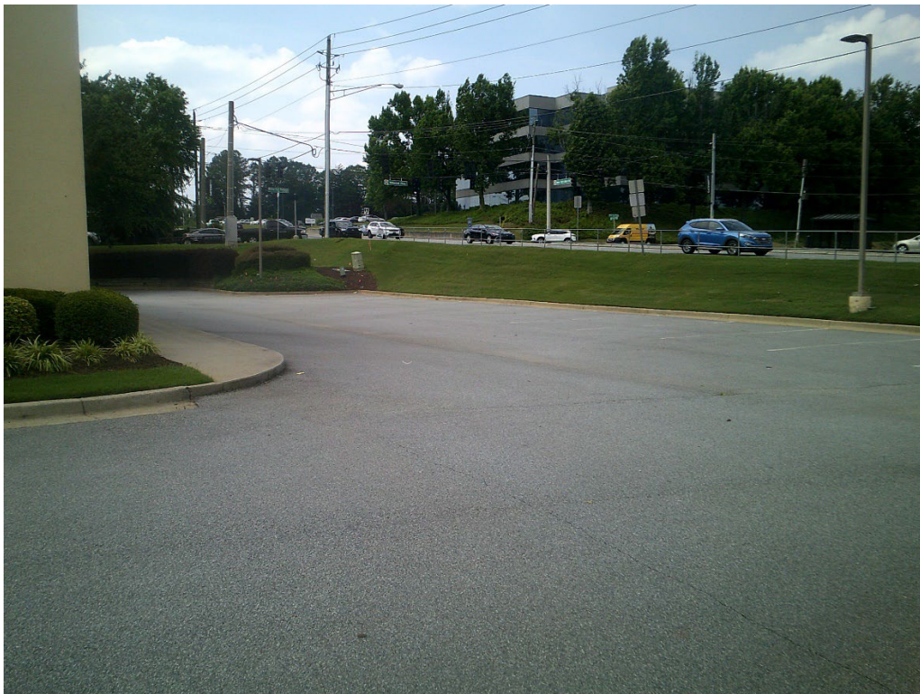
View of Existing Parking Lot
