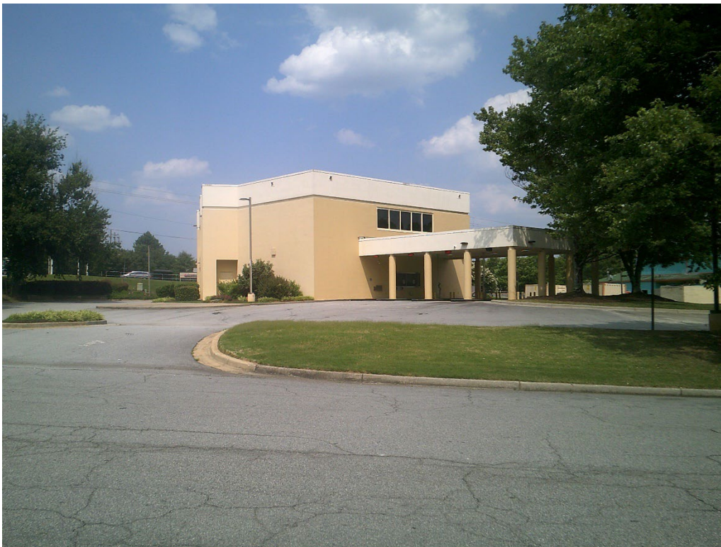
View of Existing Building from Willow Oak Trail
