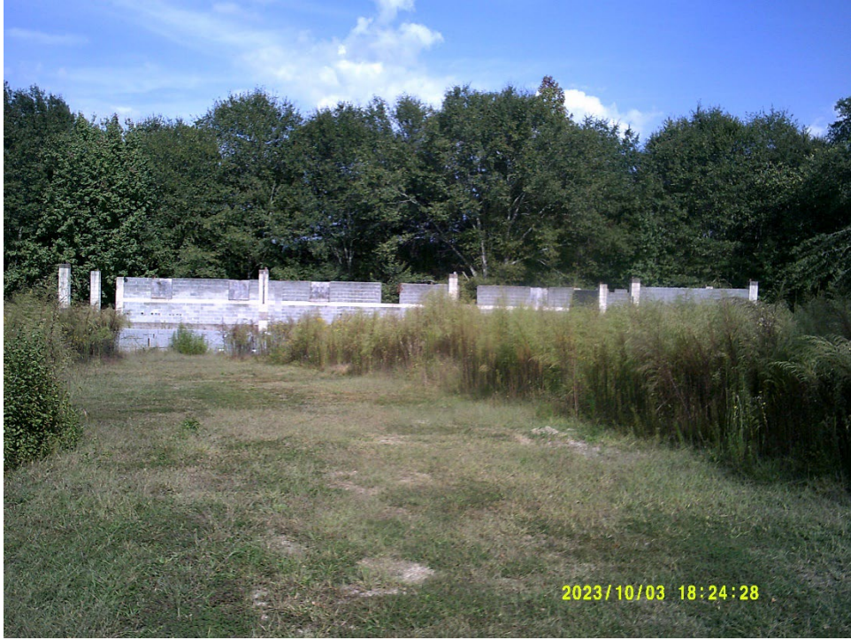
View of unfinished building in the rear
