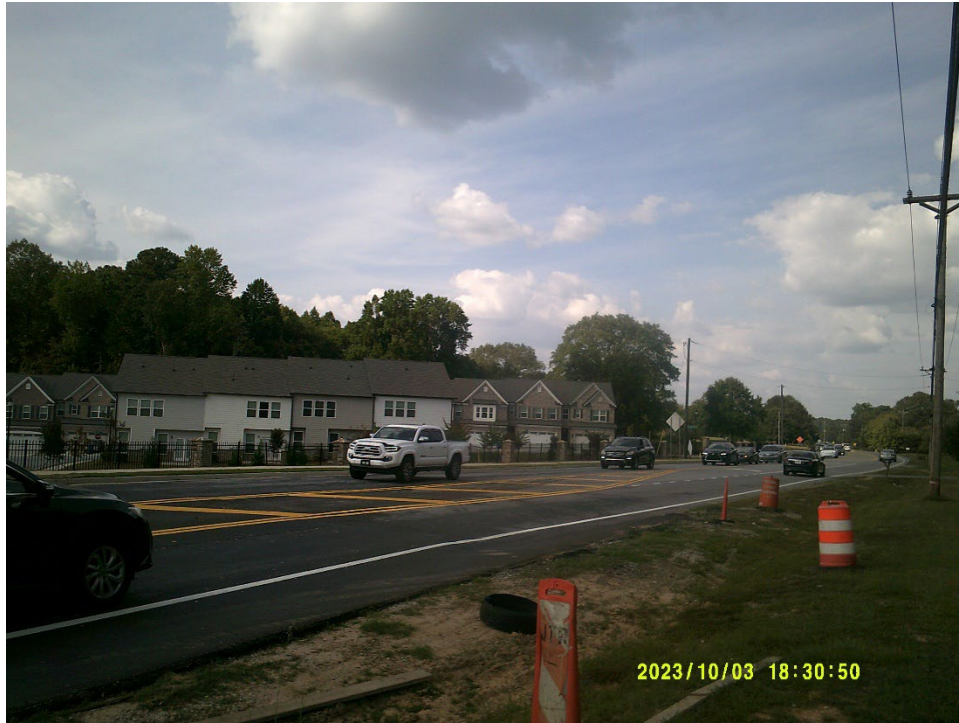
View of Rosebud Road, subject property on the right
