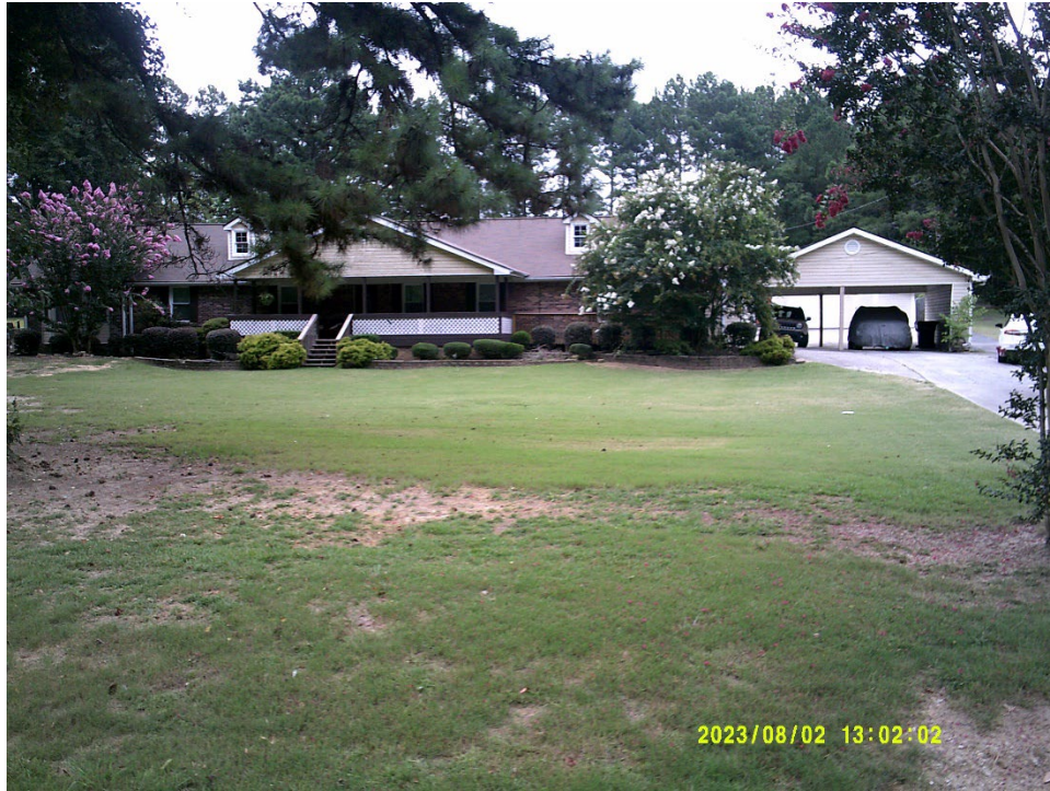
View of the Community Living Arrangement from Lee Road
