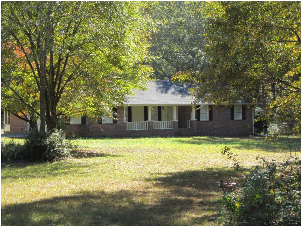
View of the existing residence
