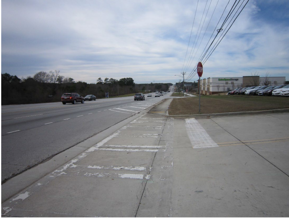
View of Athens Highway, facing west
