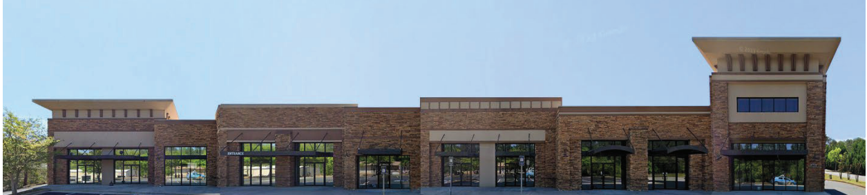
Image #1 – Main Building Elevation
