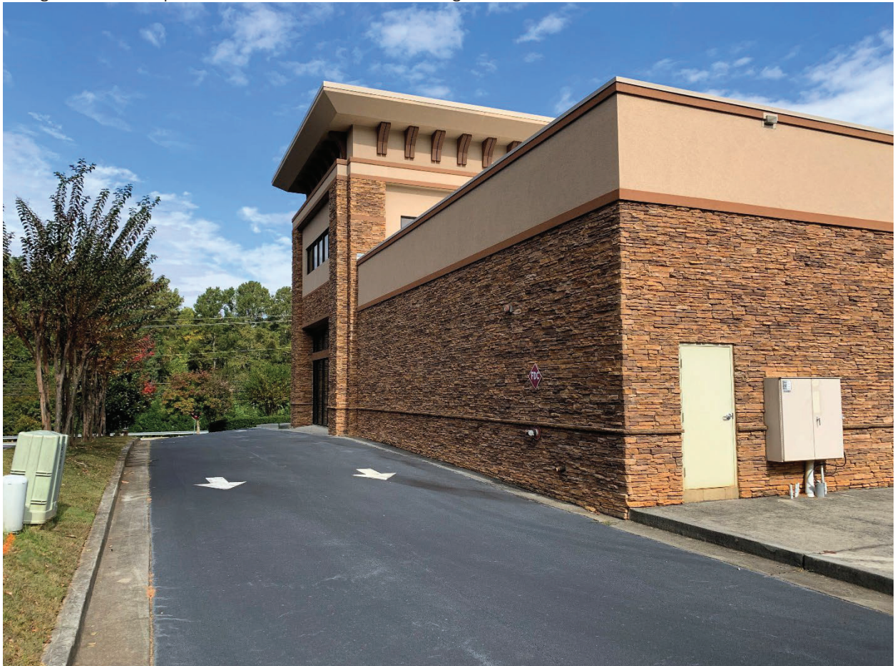
Image #8 – Perspective View of Rear of Building
