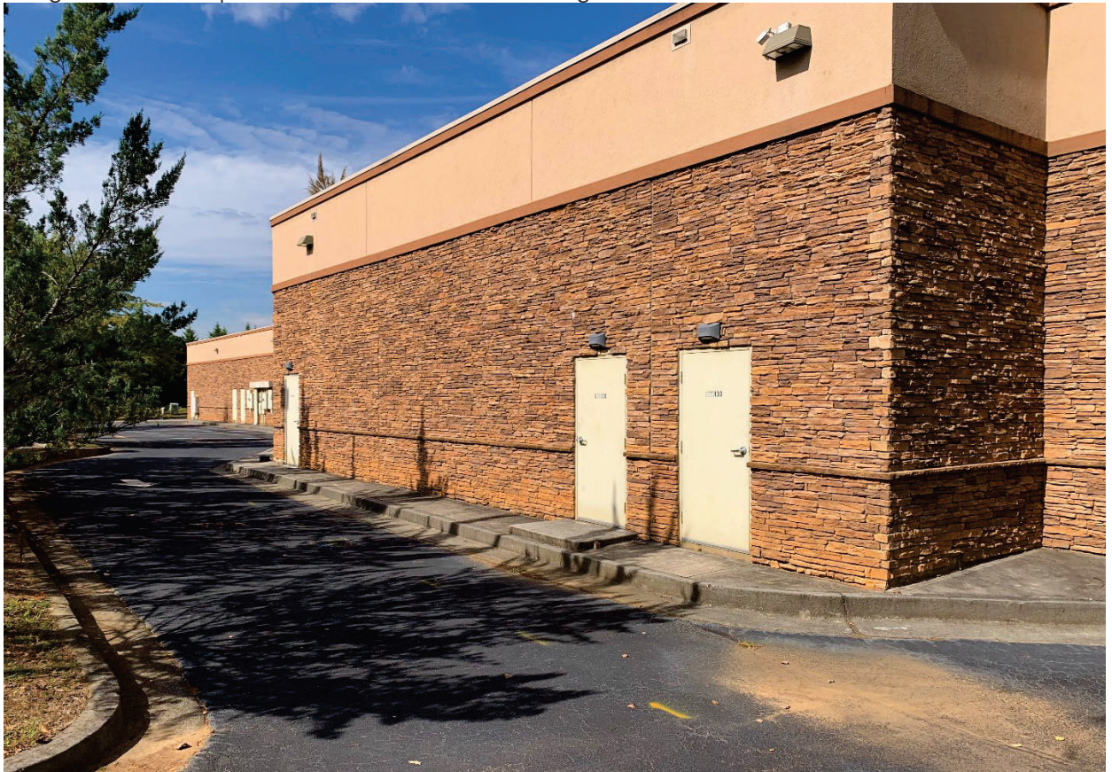
Image #10 – Perspective View of Rear of Building
