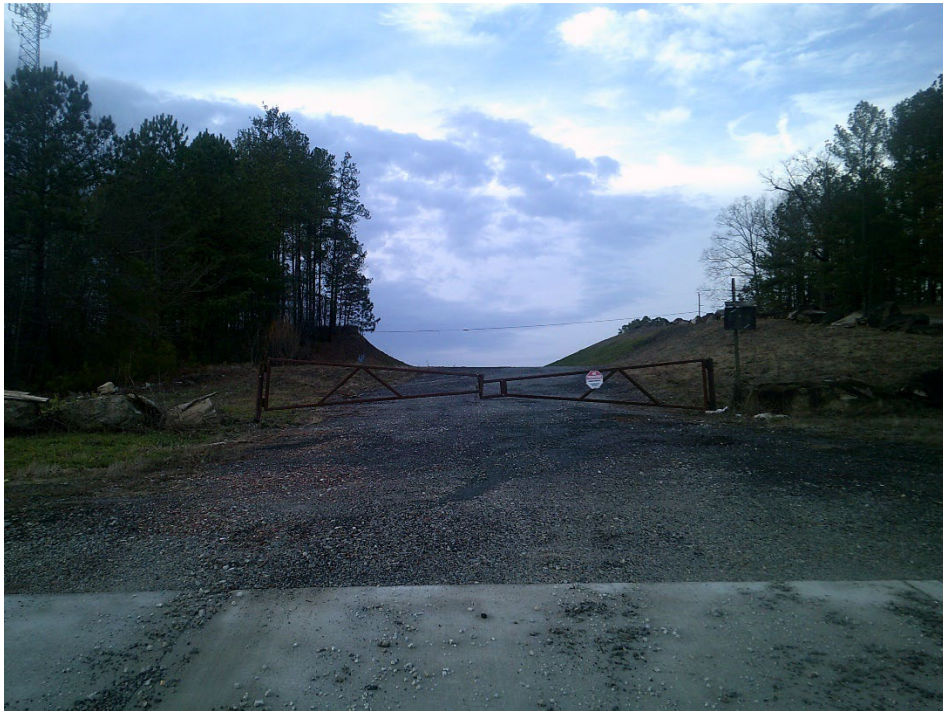
View facing north
