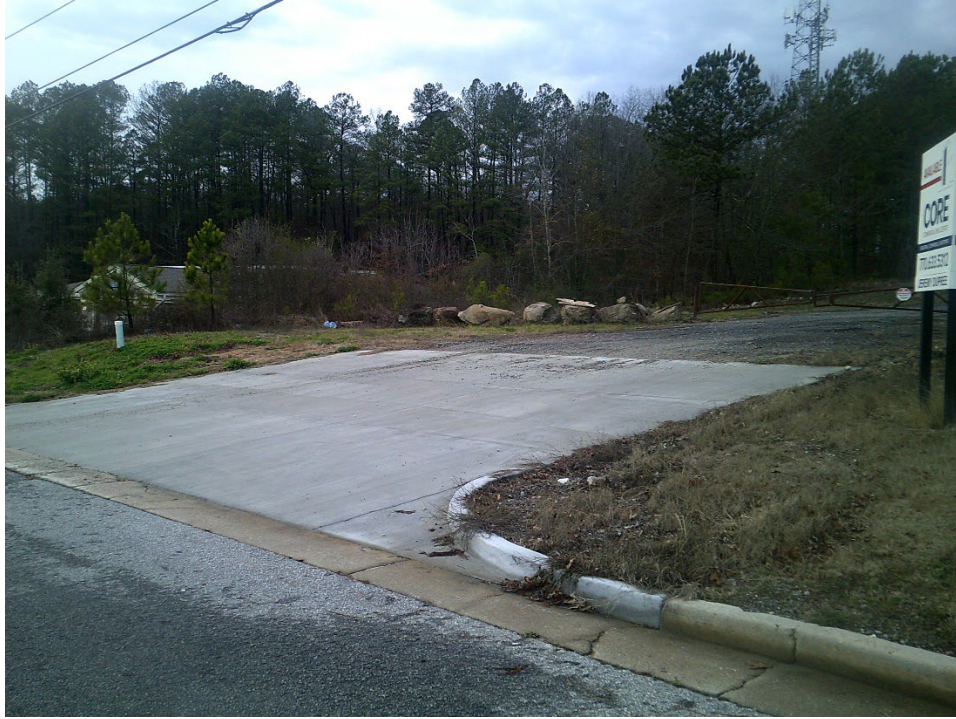
View of existing entrance to property
