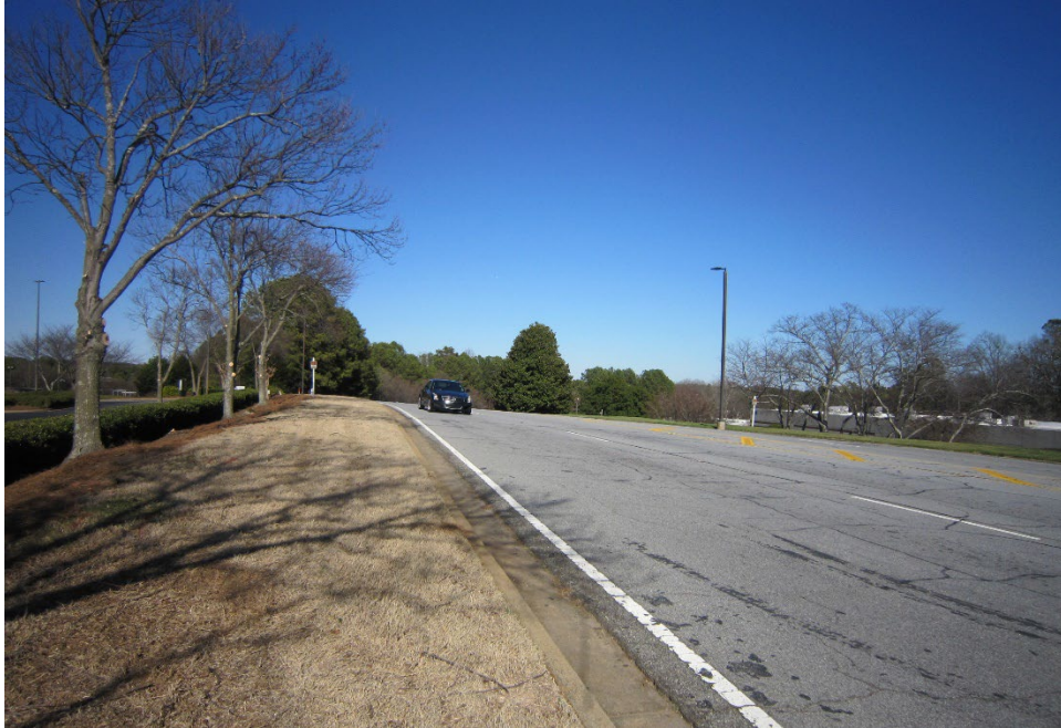
View of Breckinridge Road frontage
