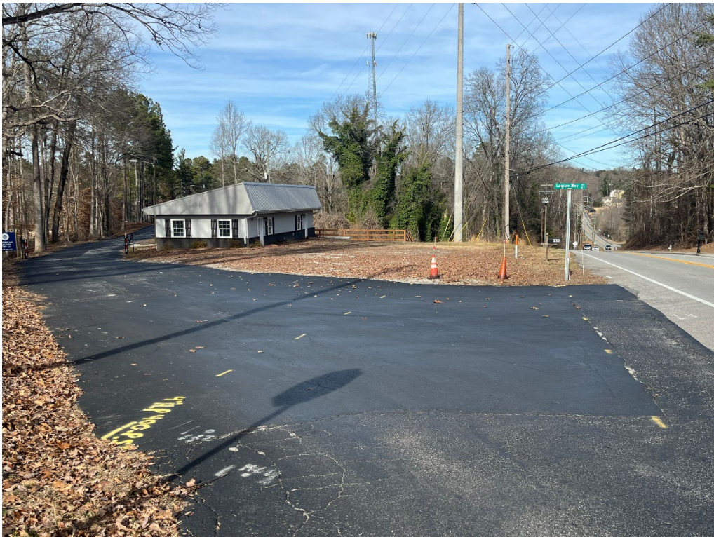
View of property facing north
