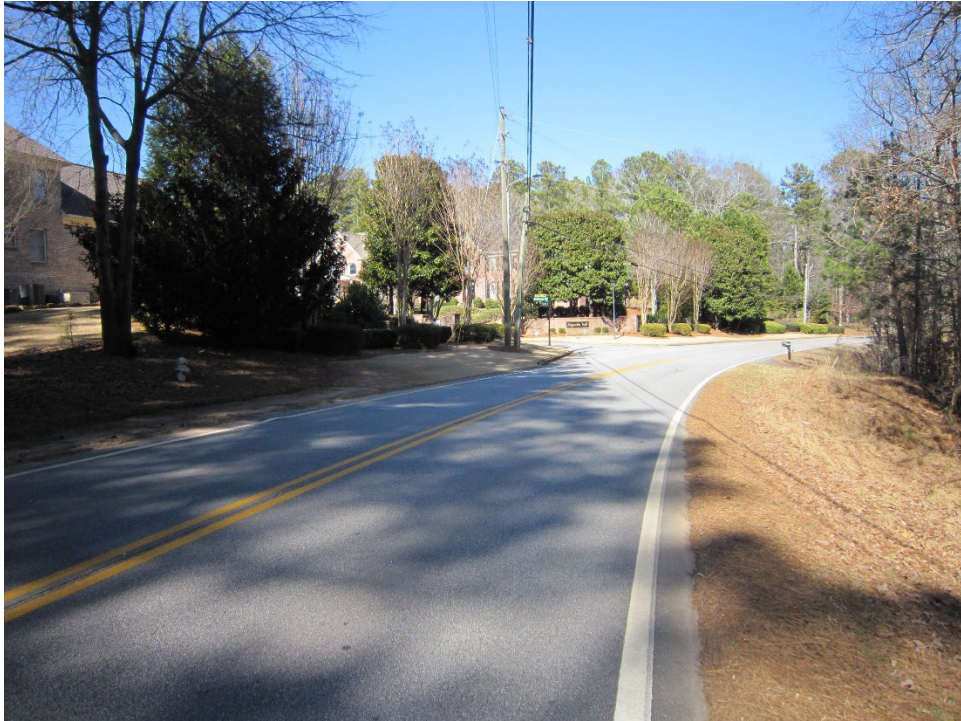
View of Wildwood Road at proposed eastern entrance, subject on right
