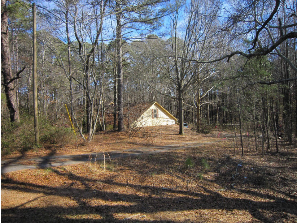
View of existing residence at 2021 Braselton Highway
