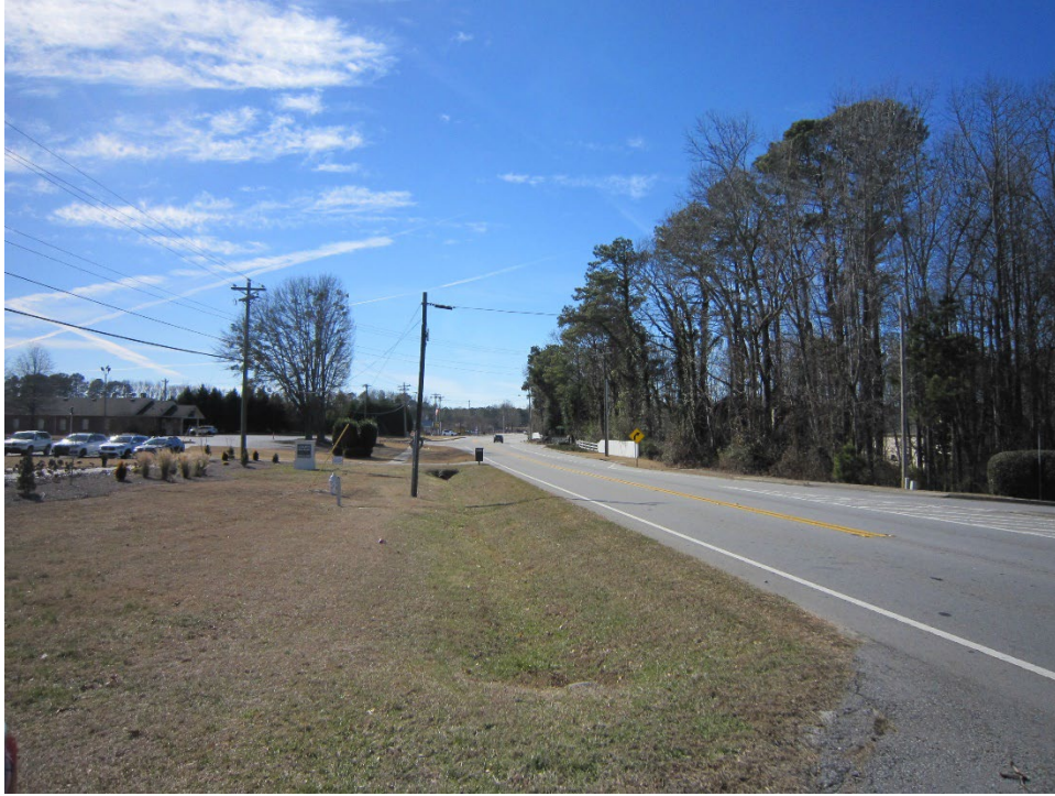
View of Braselton Highway facing west
