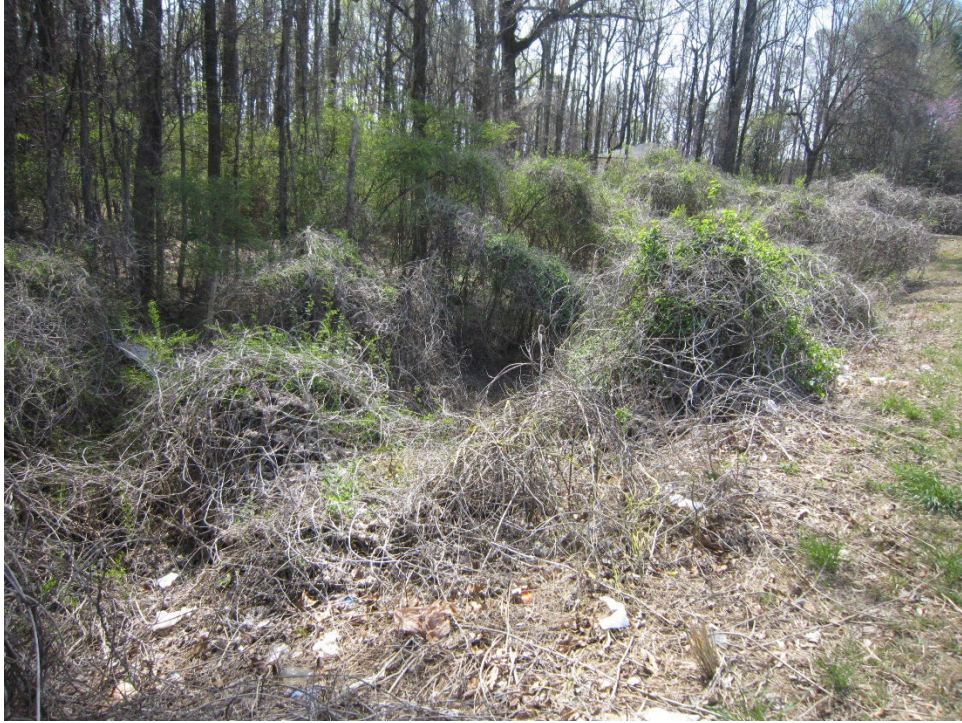
View of ditch along Lawrenceville Highway right-of-way
