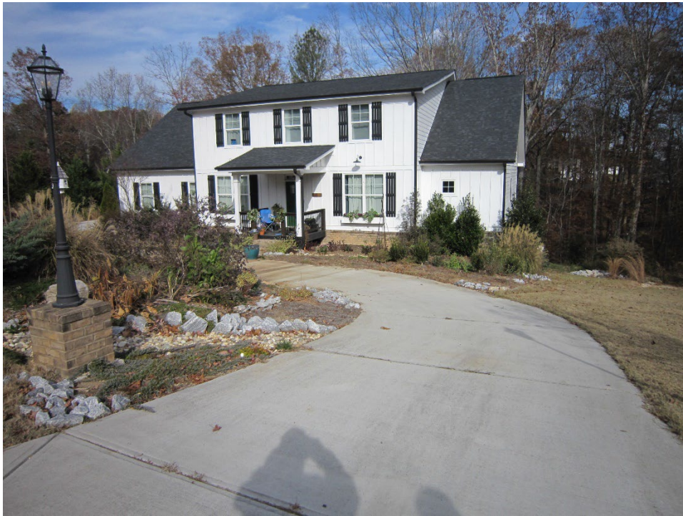
View of property across Holman Road to the north
