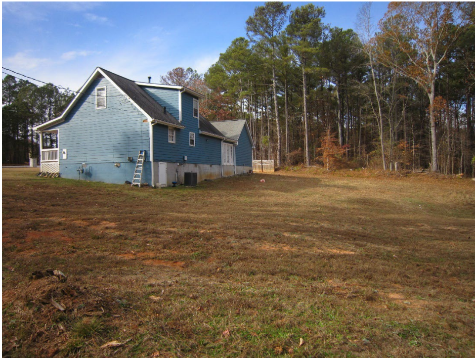
View of rear of existing residence
