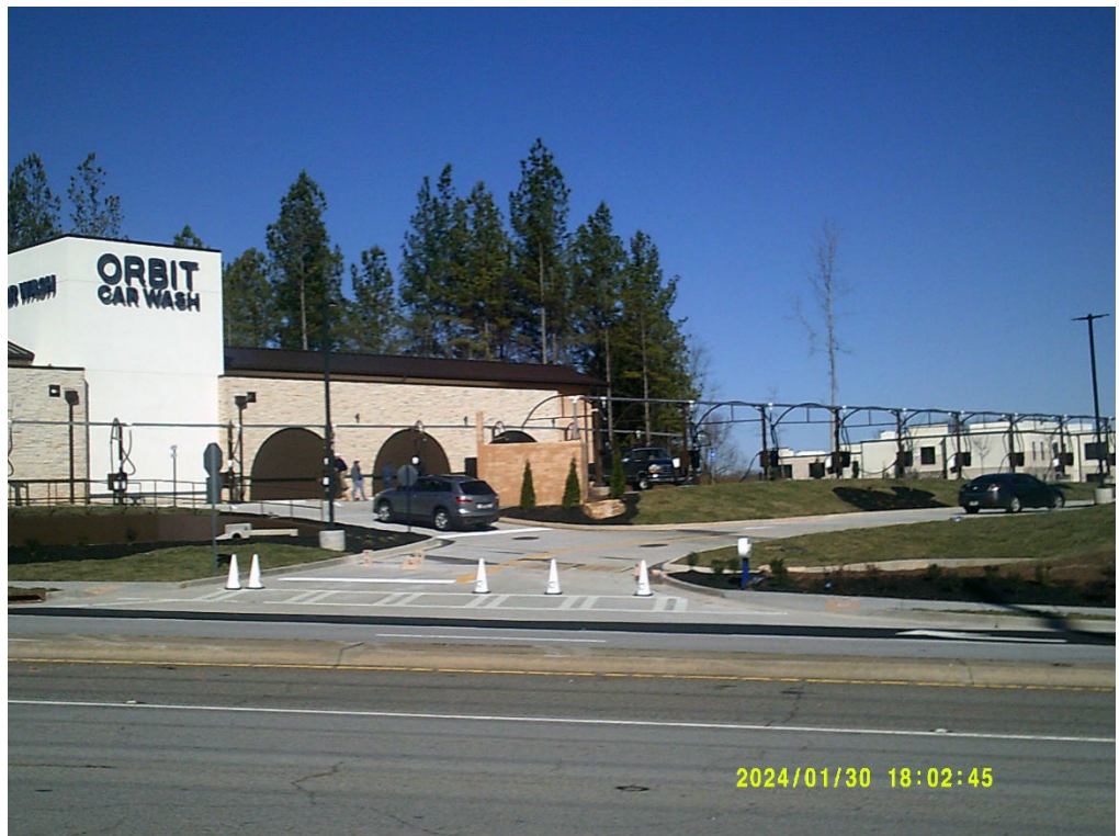
View of driveway access from Old Peachtree Road
