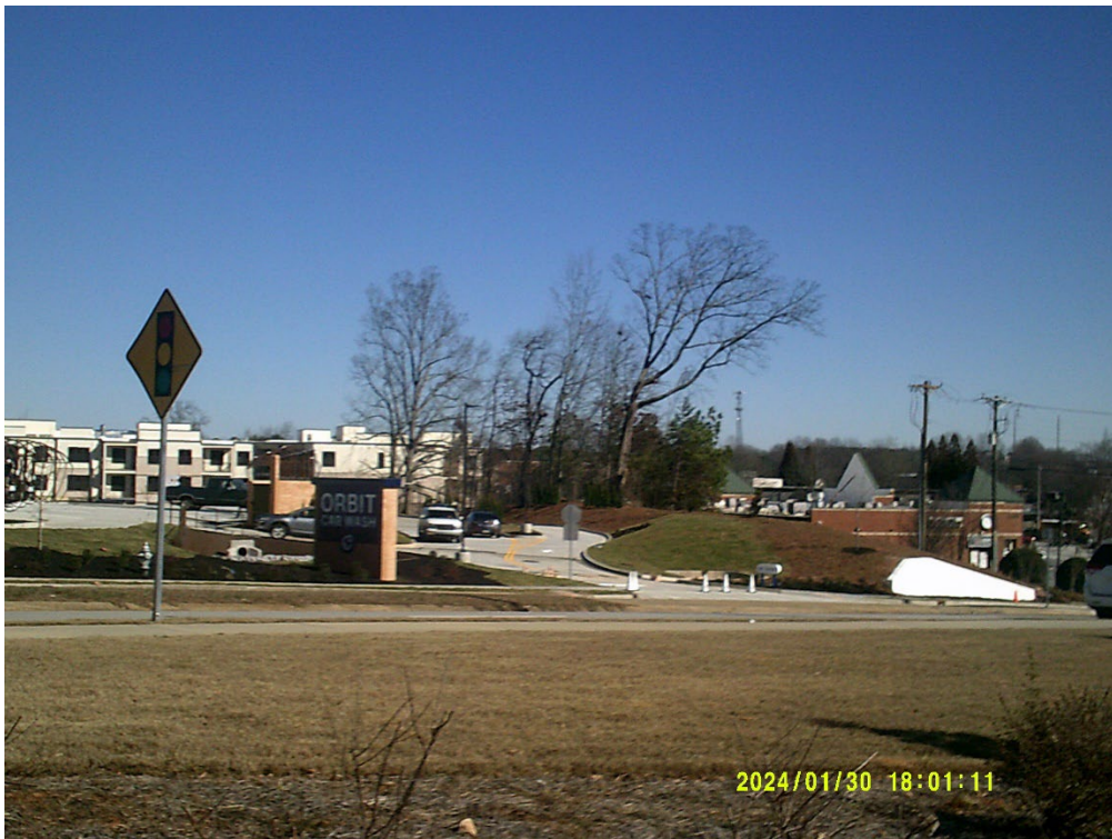
View of driveway access to the site from Old Peachtree Road
