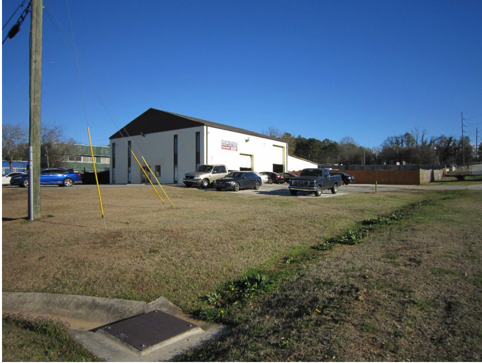
View of property from Arcado Road
