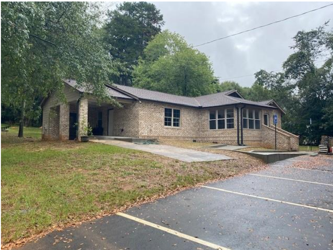
2021 conditions of the site
