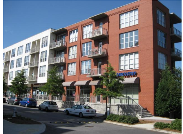
Condos above a mix of service and commercial uses including a dentist and small gym are supported by pedestrian oriented environment with on-street parking, street trees, and a lower level parking deck.
