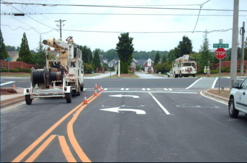
US 78 / SR 10 / Main Street at Abington Drive
