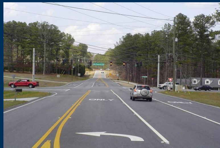
Old Fountain Road at Old Peachtree Road
