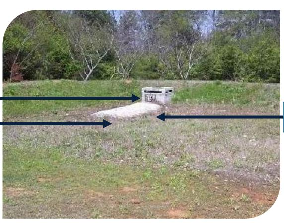
Channel Protection with Trash Rack
