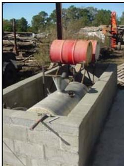
Cinder block secondary containment on slab with roof
