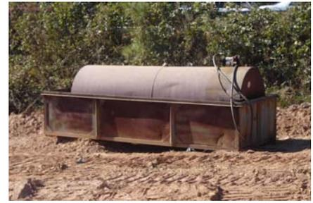
Improper storage of fuel on construction sites will increase the risk of water pollution that may occur as a result of leaks or spills.
