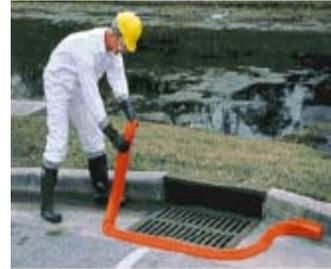
Berms may also be used to assist in directing washwater to a predetermined collection area. Inexpensive “Pool Cover Water Tubes” available from pool supply stores can be used for this purpose. These berms may not form a water tight seal against the ground and as such may not be suitable as a protective barrier around a storm drain.
