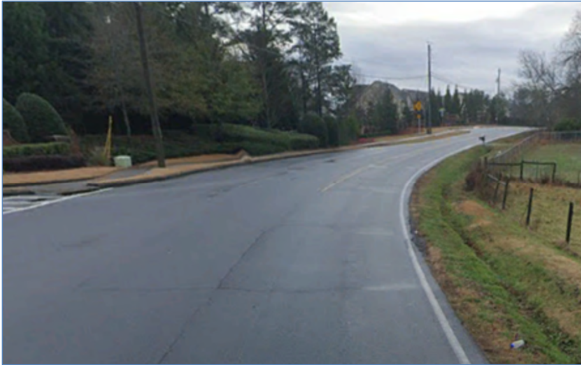
Kilgore Road & Access - looking south
