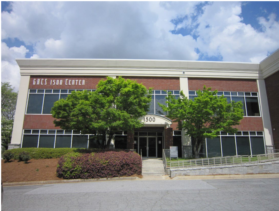
View of 1500 Center building located across Indian Trail-Lilburn Road
