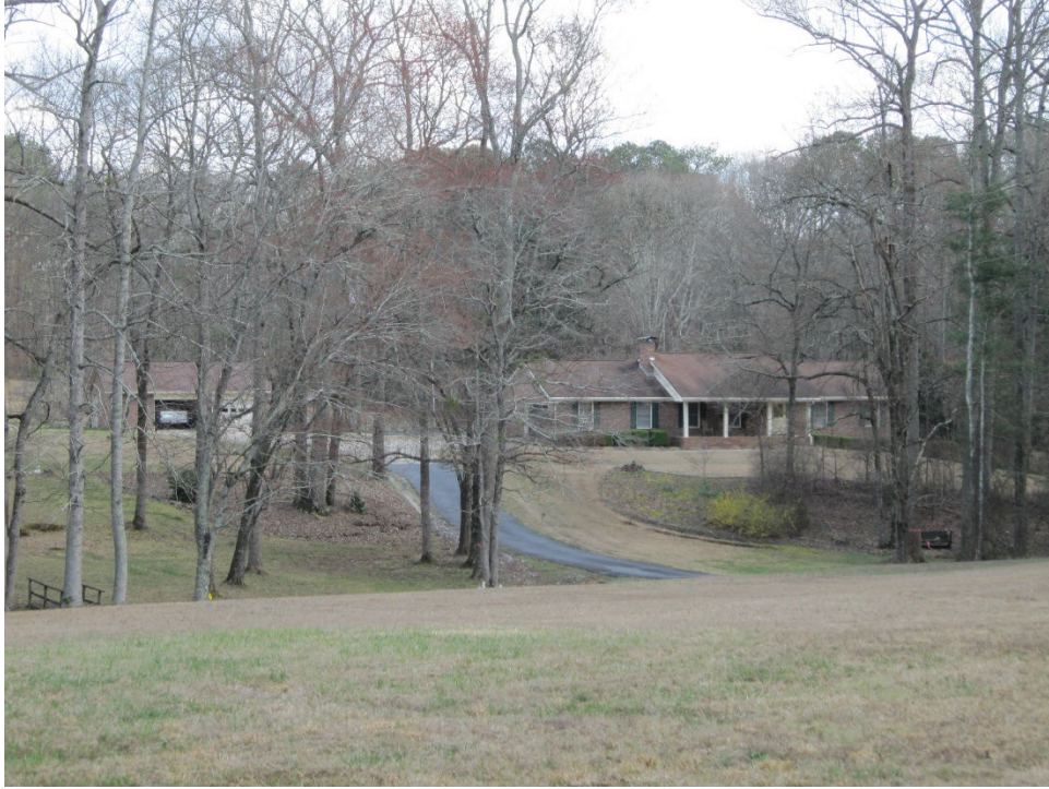
View of second existing residence on the site
