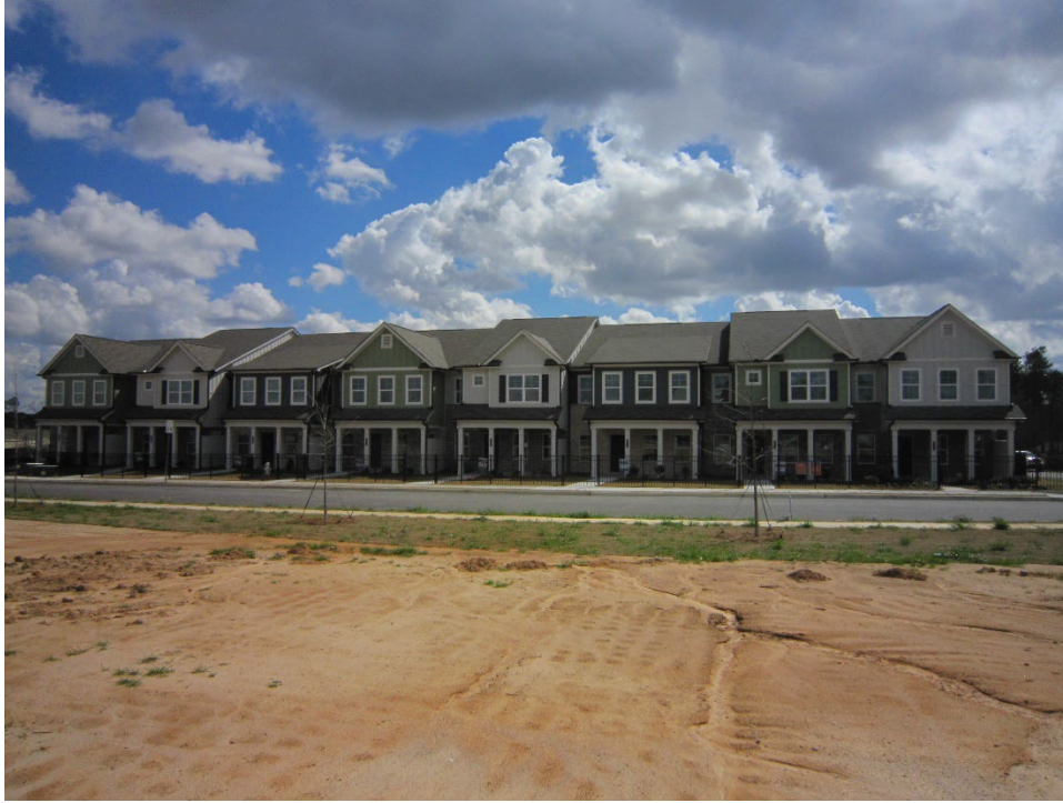
Front façade of existing townhouses
