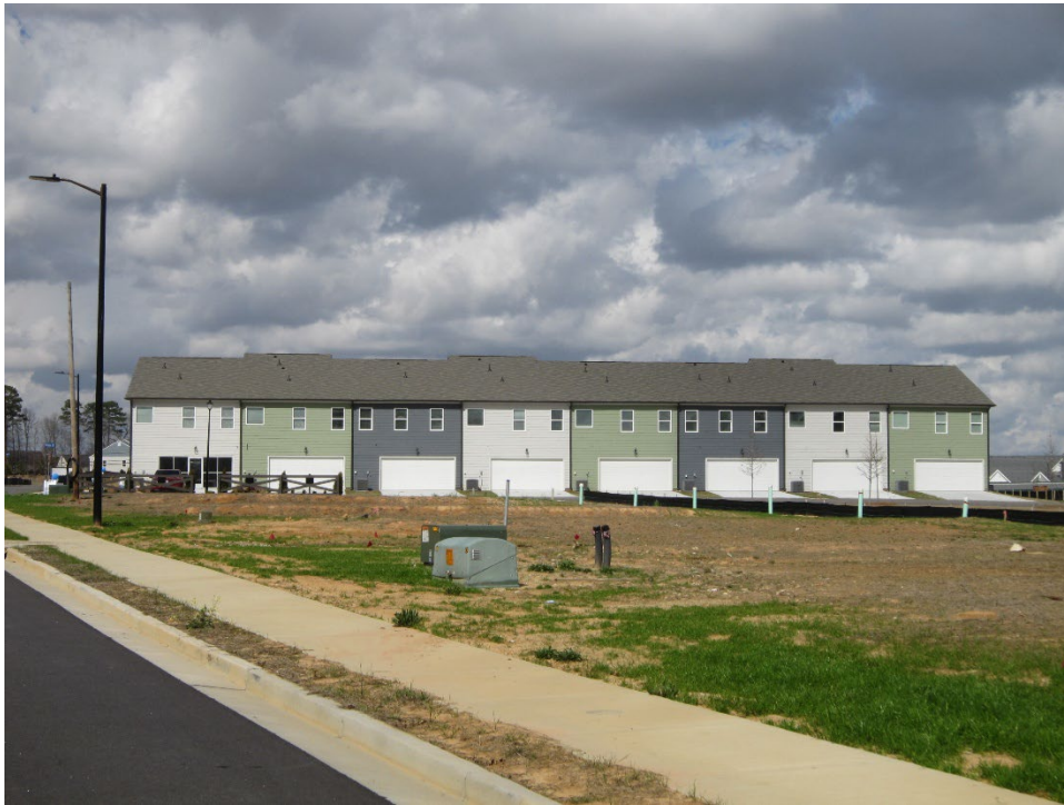
Rear façade of existing townhouses
