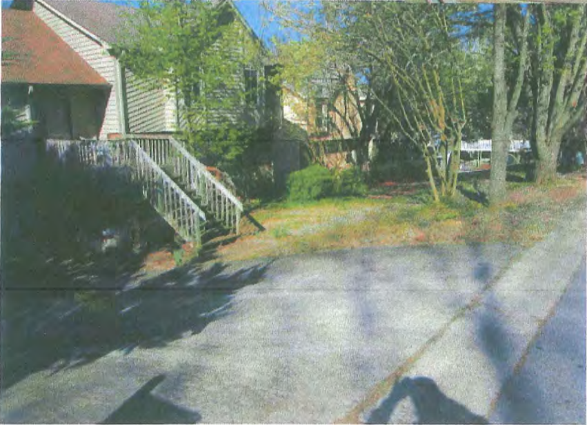
VIEW OF DECK FROM STREET
