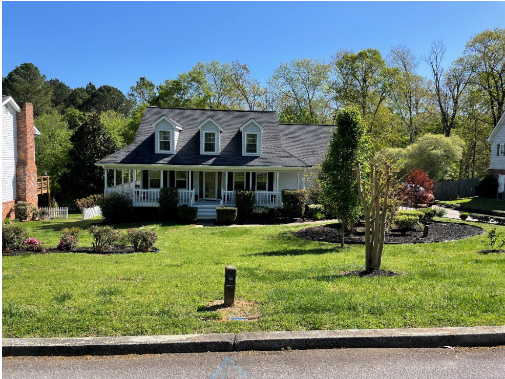
Photo Facing Front Façade of Building
