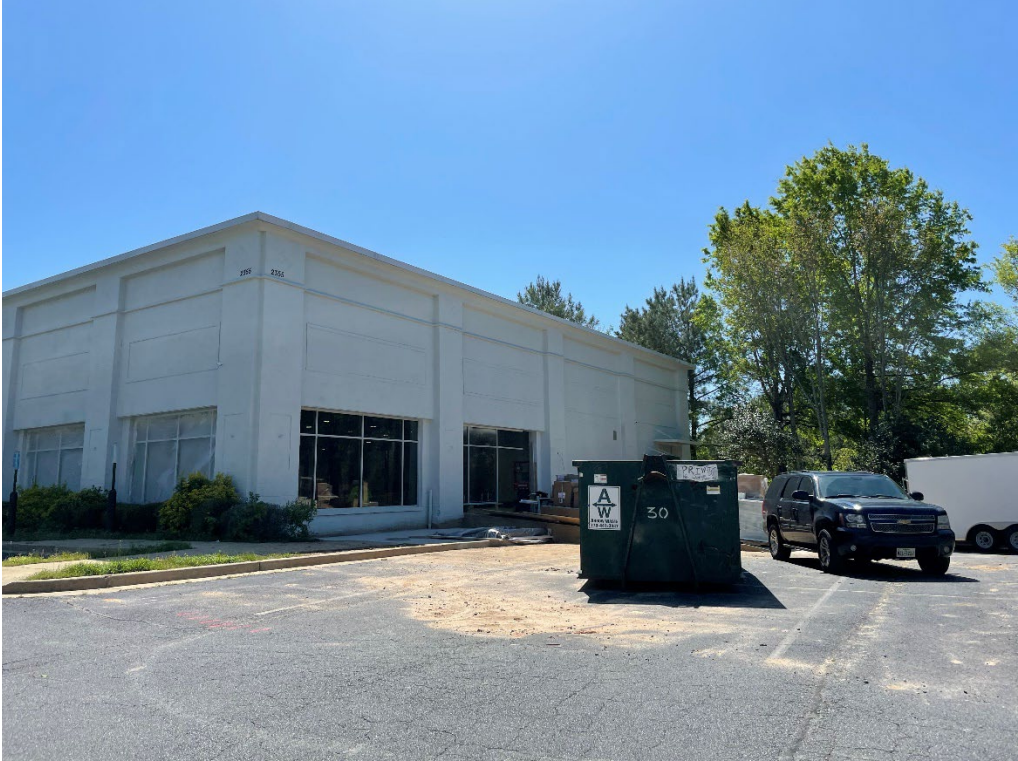
View of West Elevation
