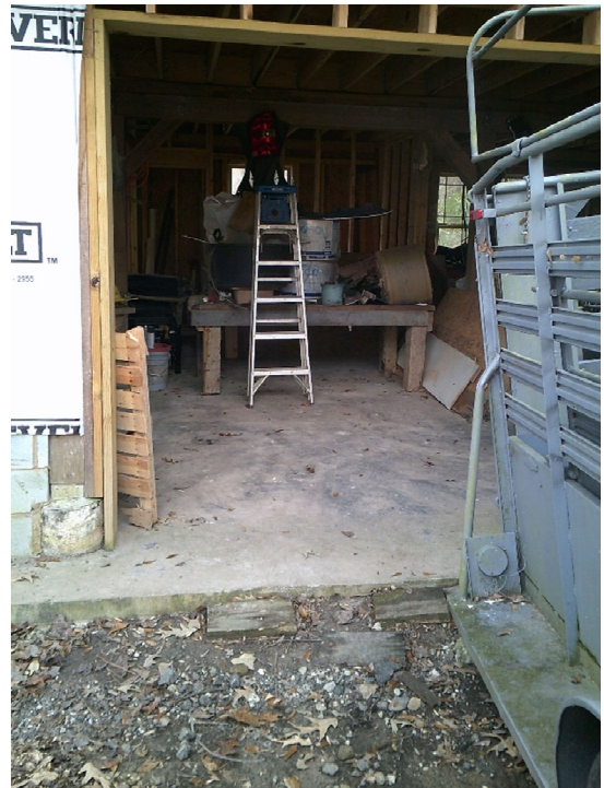
Accessory Dwelling Northern Side with Ground Floor Storage (Facing Principal Housing Structure)
