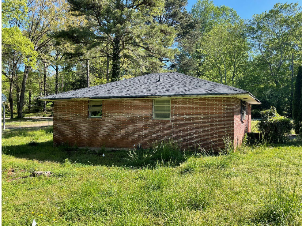
Photo Facing Western Façade of Accessory Building
