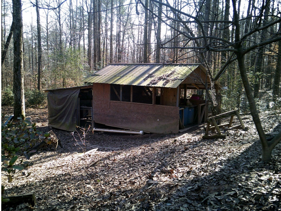
Shed to be Removed
