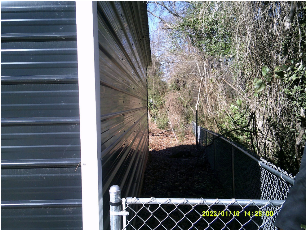
Accessory Building Rear View (Adjacent to Property Line)
