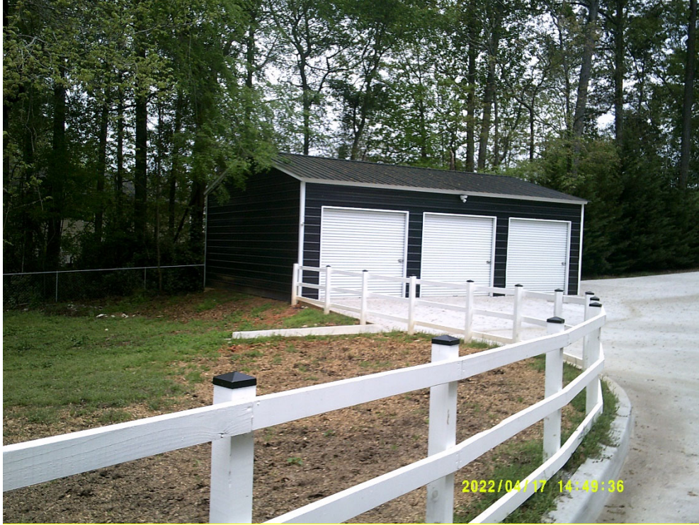
Accessory Building Front View
