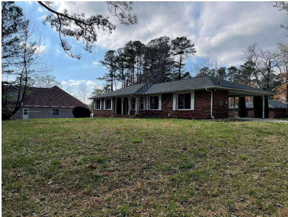
Photo Facing Northwest showing Carport
