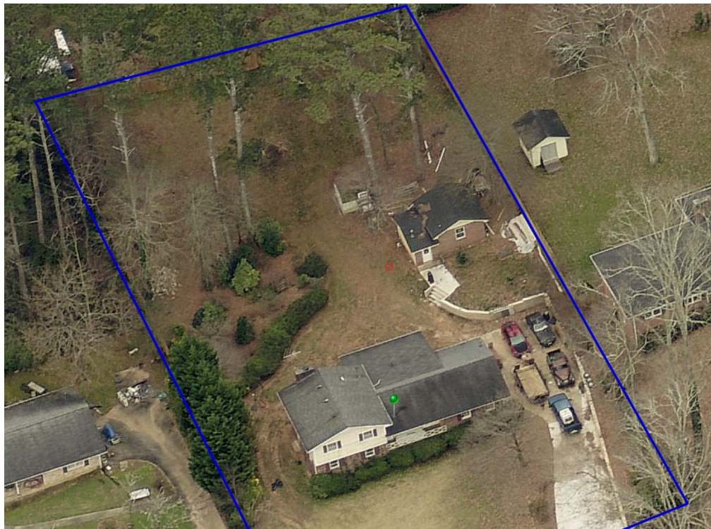
Aerial imagery of principal structure and existing accessory structure
