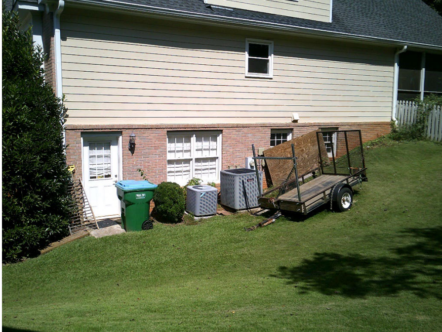
Side entrance for wheelchair accessibility
