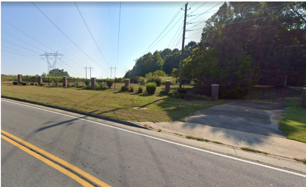
Power Easement on northern portion of property
