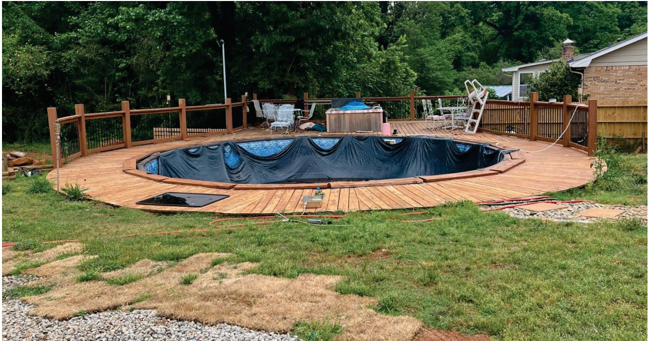
View of wooden pool deck
