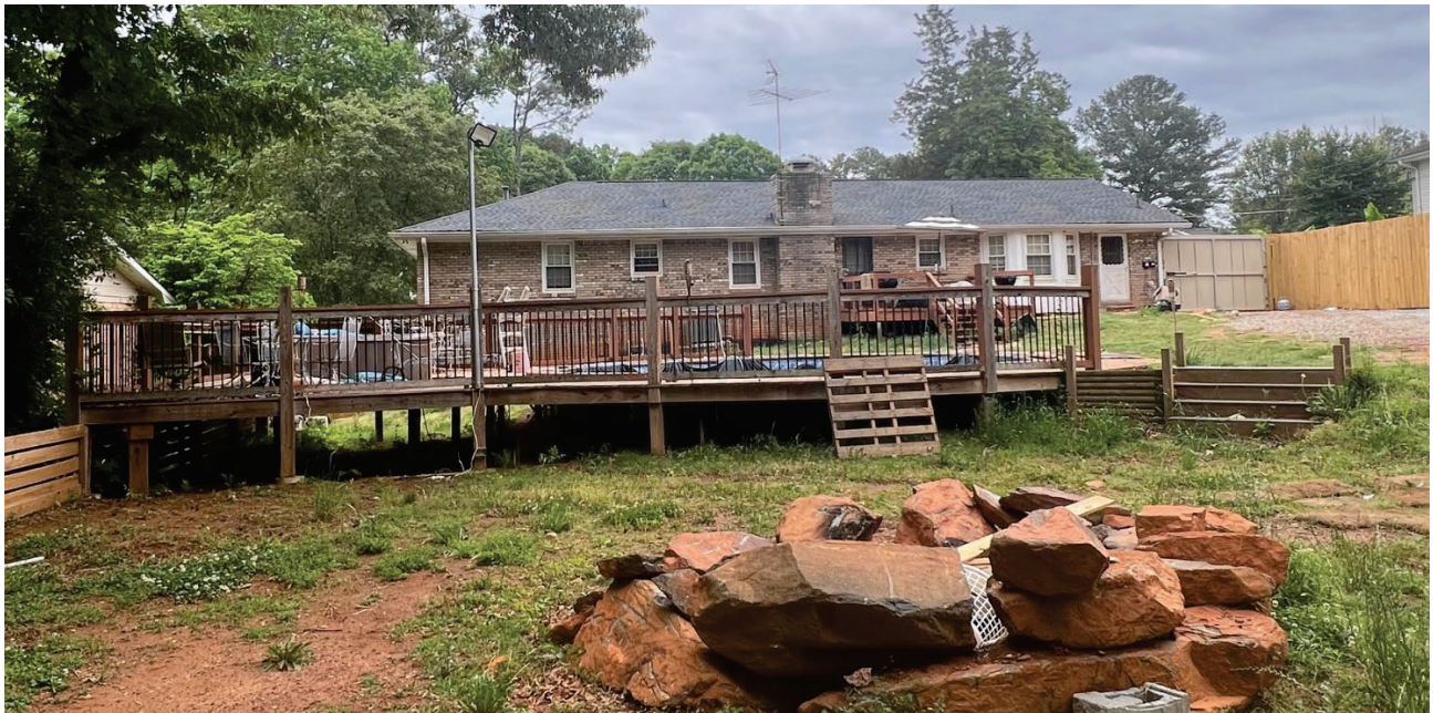
View of wooden pool deck
