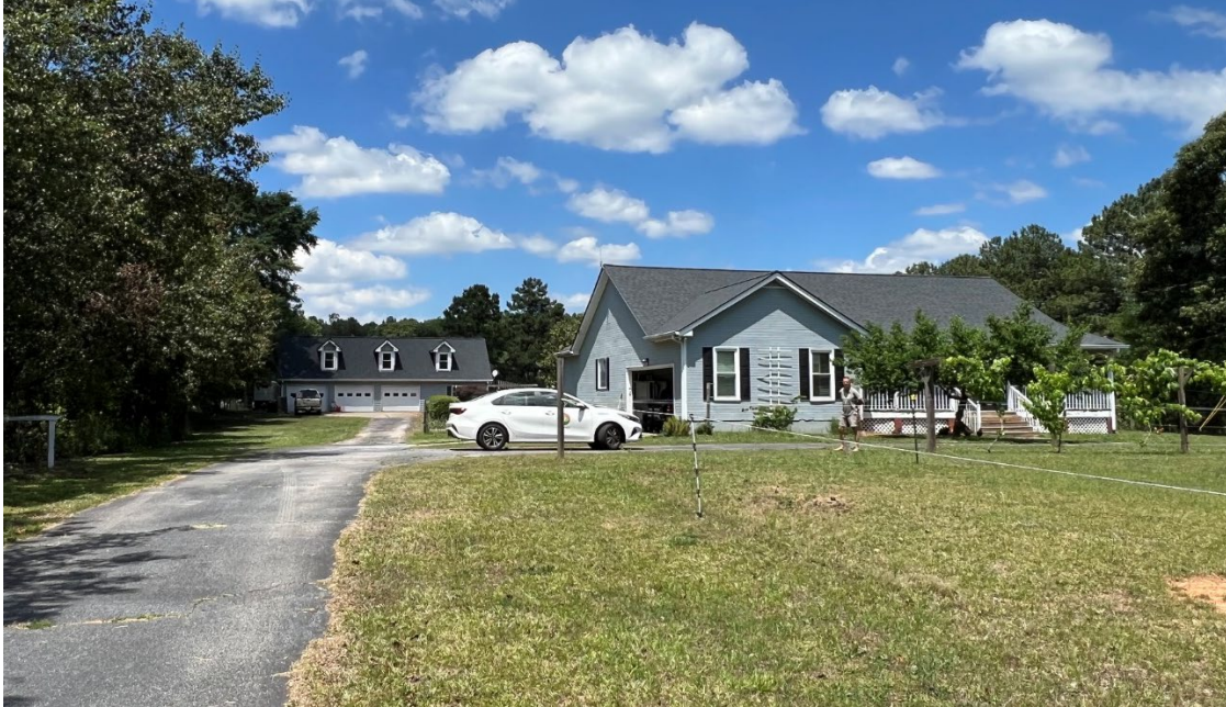
View of property from driveway
