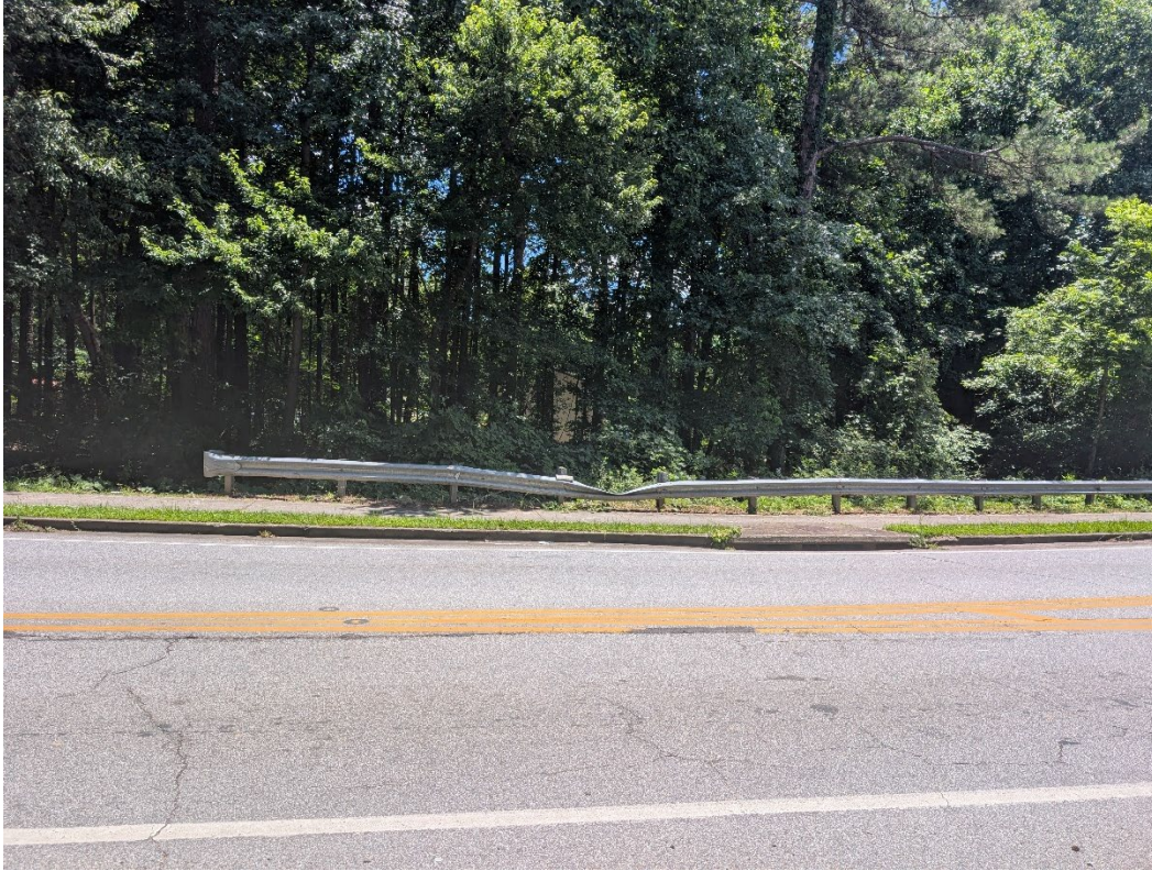
View from Williams Road
