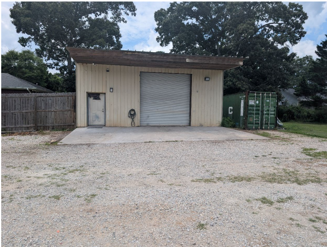
Rear façade of Building A
