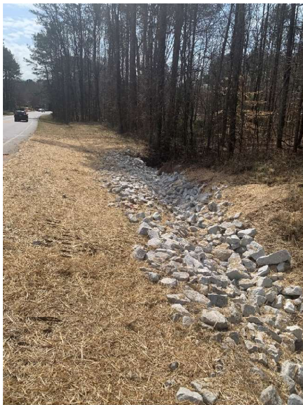
Figure 1-9. Approx. Right of Way Stream Entry onto Site, Looking South Post RipRap Install
