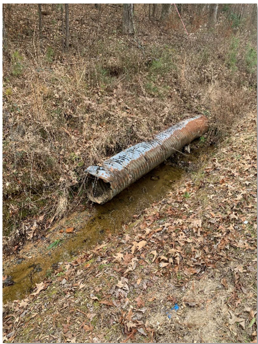
Figure 1-7. Eroded Culvert in Unnamed Trib.
