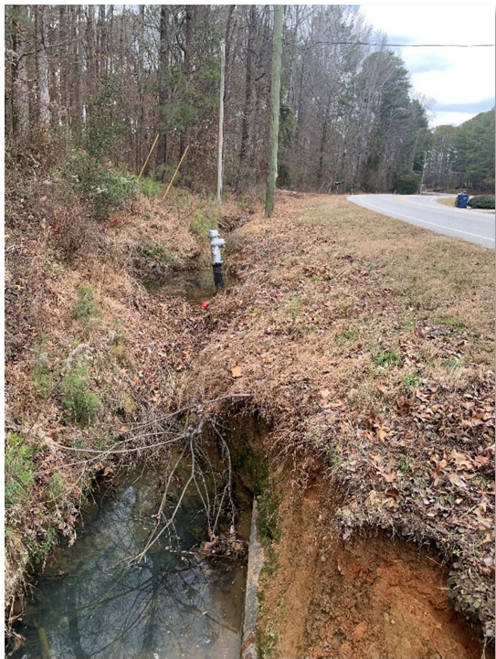
Figure 1-5. Upstream Extent of Unnamed Trib. Eroding Water Line (Looking North on West Side of Mink Livsey)
