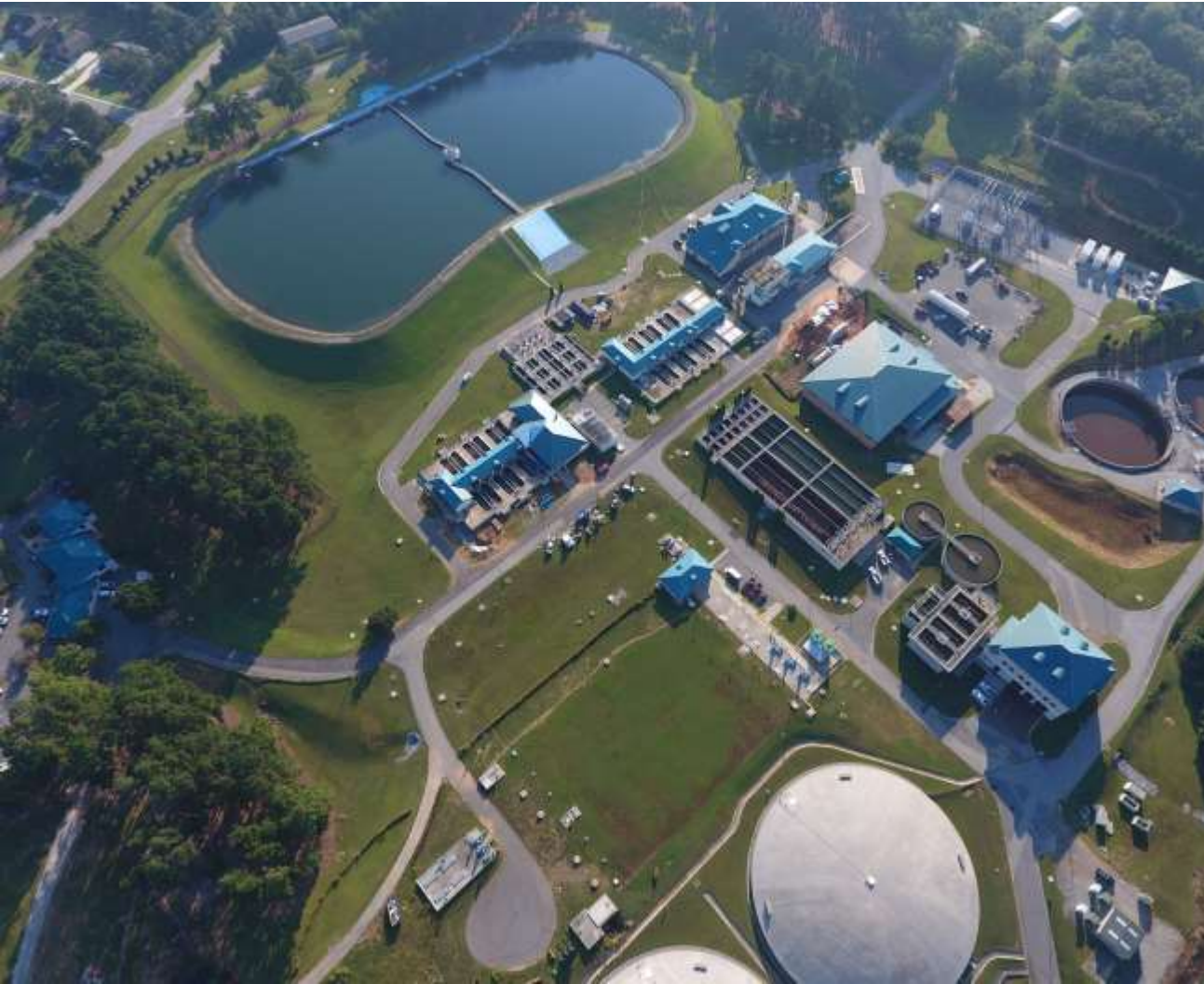
Water Production Facilities
