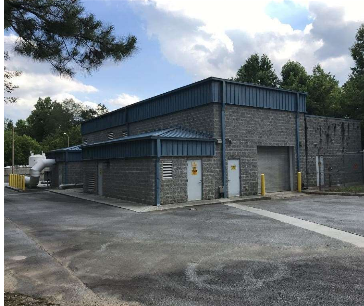
Wastewater Pump Stations
