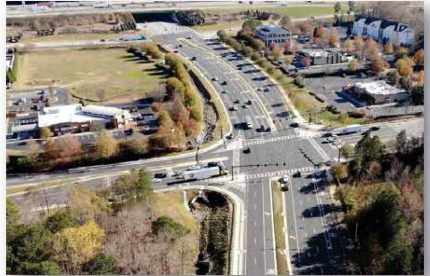
Sugarloaf Parkway at Satellite Boulevard
