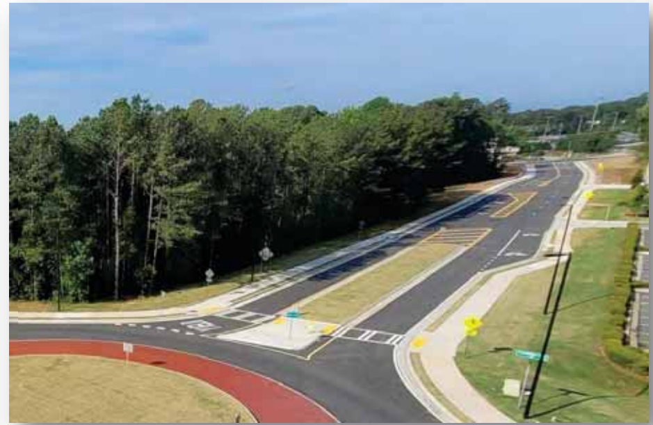
Nash Street Extension City of Lawrenceville Managed Project
