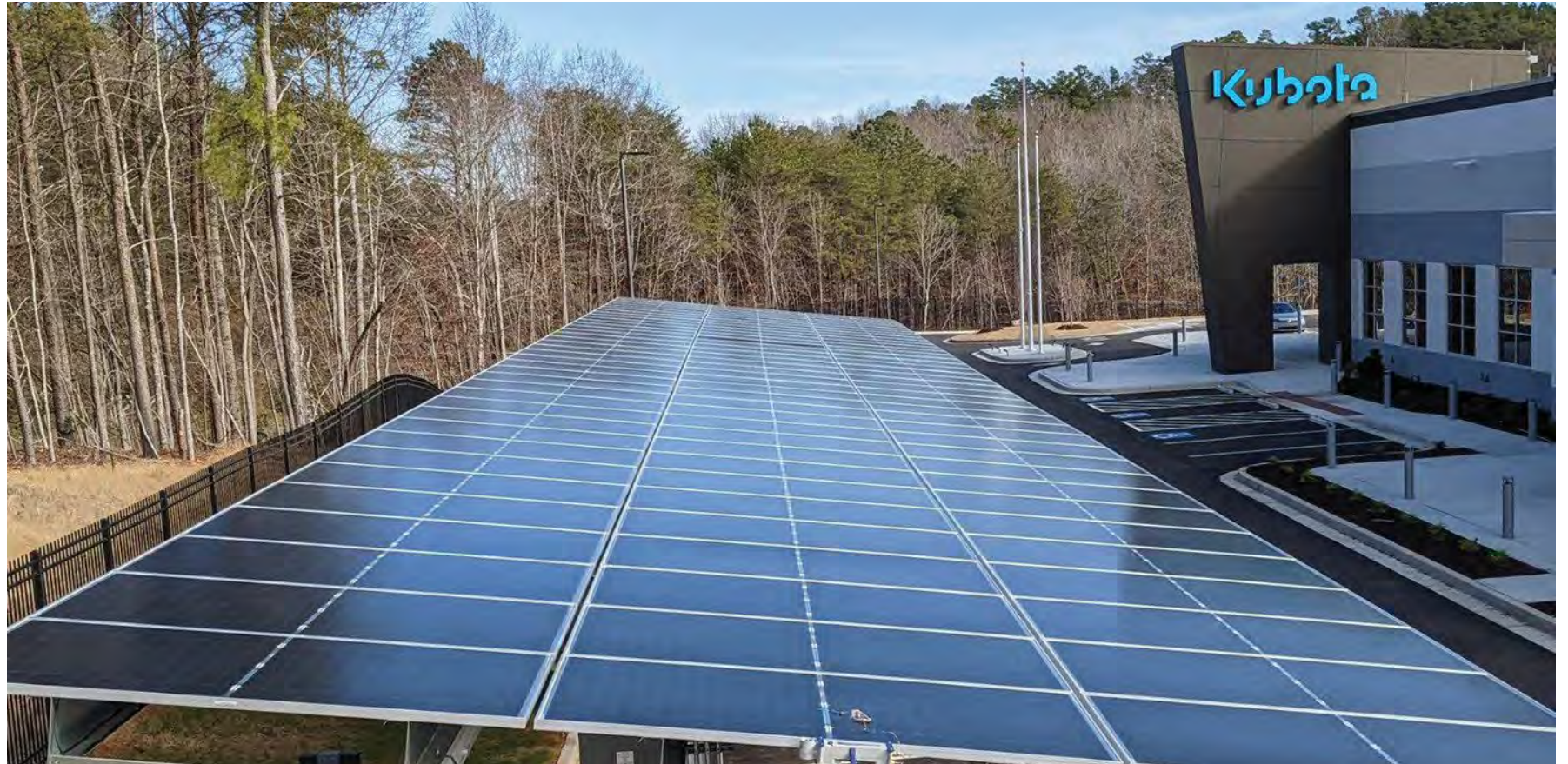
Kubota Research & Development North America Facility, Gainesville, GA
