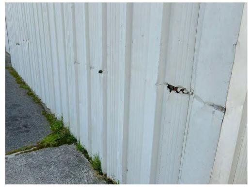
**Photograph 14.**Detail of damage to metal siding
