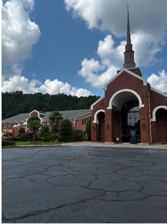
View of main building
