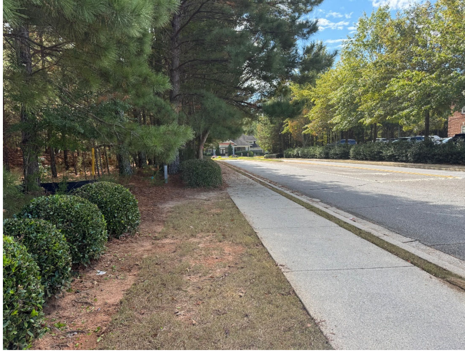
View of 5-foot-wide sidewalk along Street Frontage
