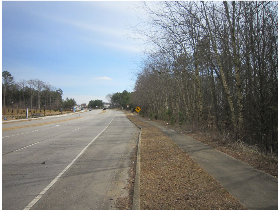
View of site frontage and shoulder along McGinnis Ferry Road
