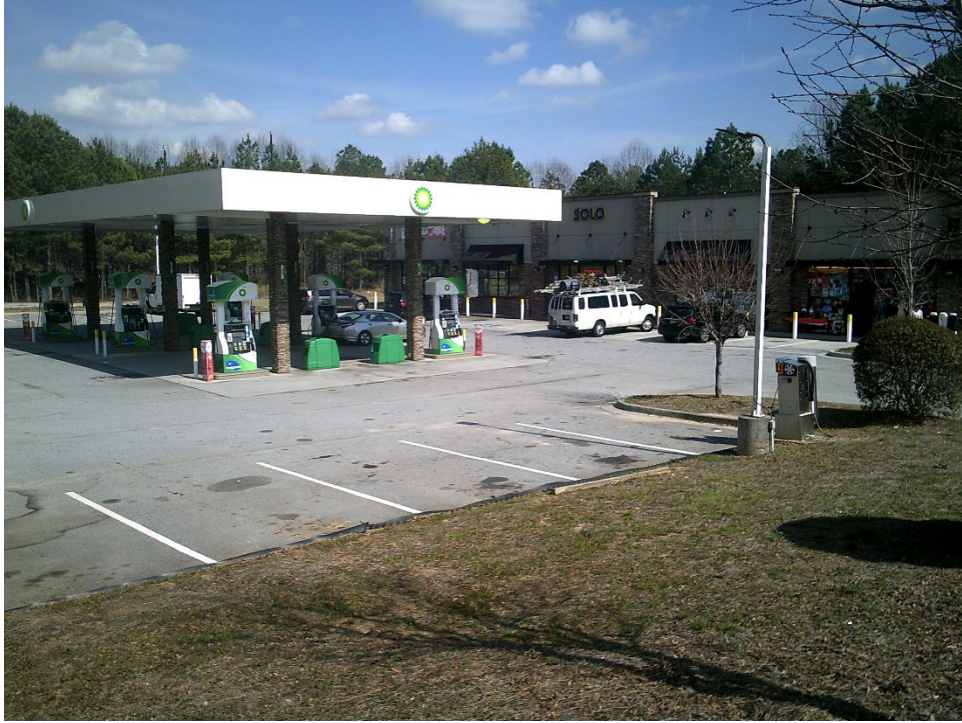
Adjacent convenience store, with fuel pumps
