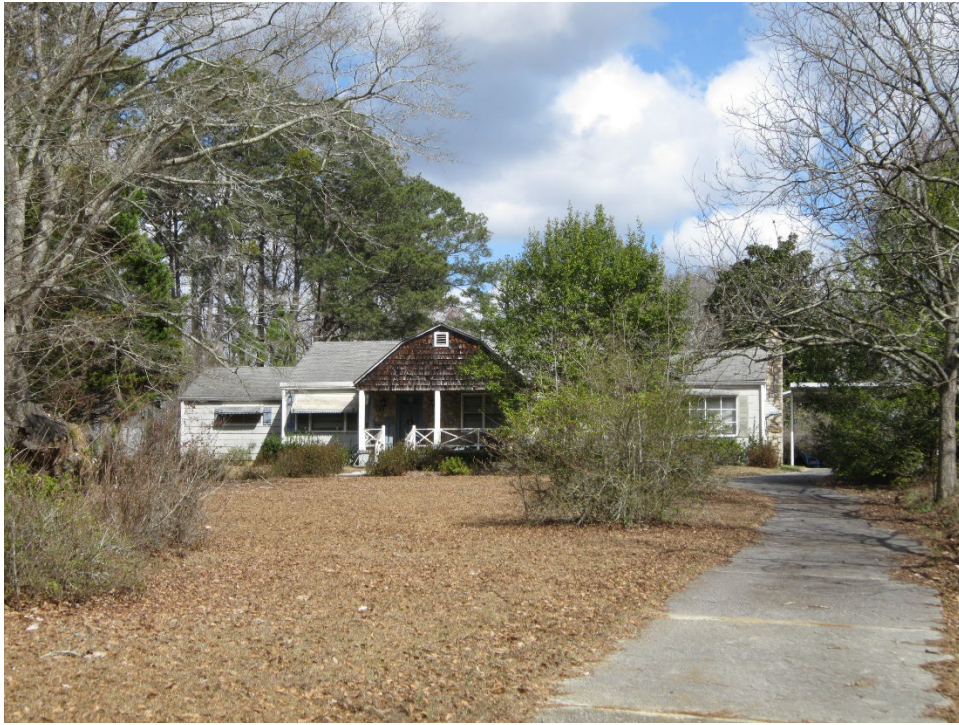
View of existing residence on site
