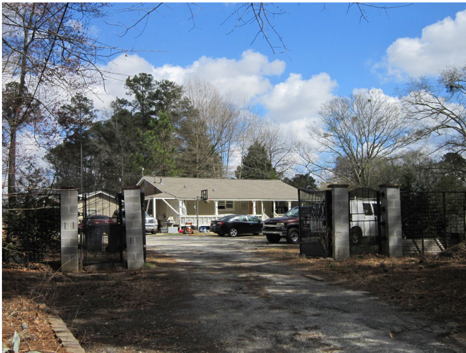
View of existing residence on site
