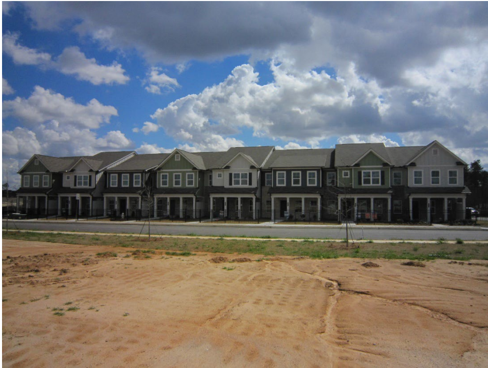
Front façade of existing townhouses
