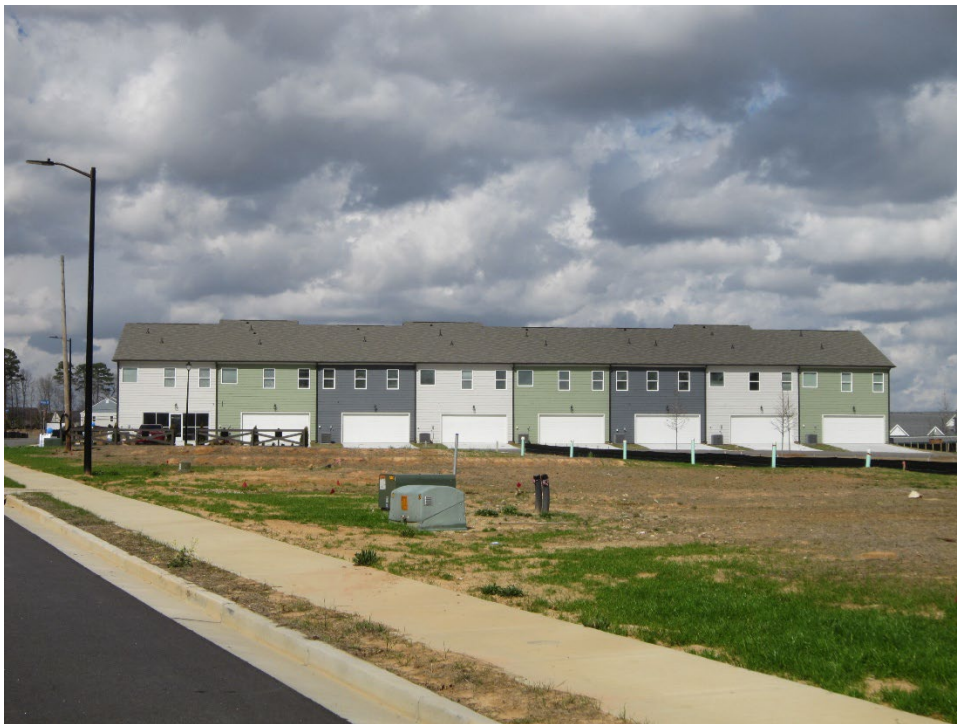
Rear façade of existing townhouses
