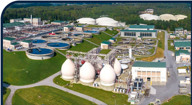
Water and Wastewater Utility
