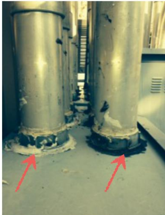
Photograph No. 5: EC-04-01 through 03: Roof (Gray Caulk) EC-05-01 through 03: Roof (White Caulk) No Asbestos Detected
