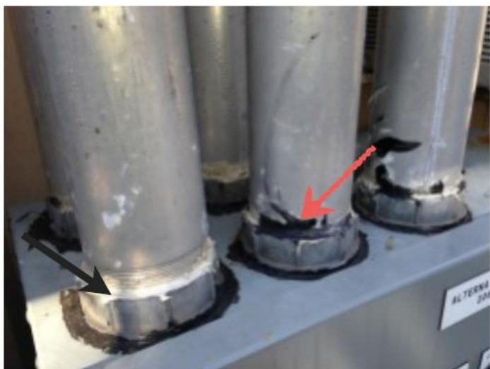
Photograph No. 3: EC-01-01 through 03: Pipes on East Wall (White Caulk) EC-02-01 through 03: Pipes on East Wall (Black Caulk) No Asbestos Detected
