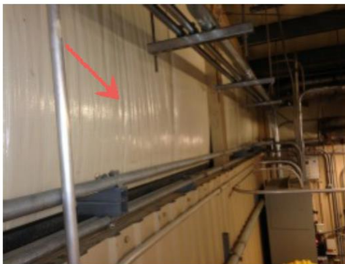
Photograph No. 2: WS-01-01 through 03: All Upper Wall Systems No Asbestos Detected
