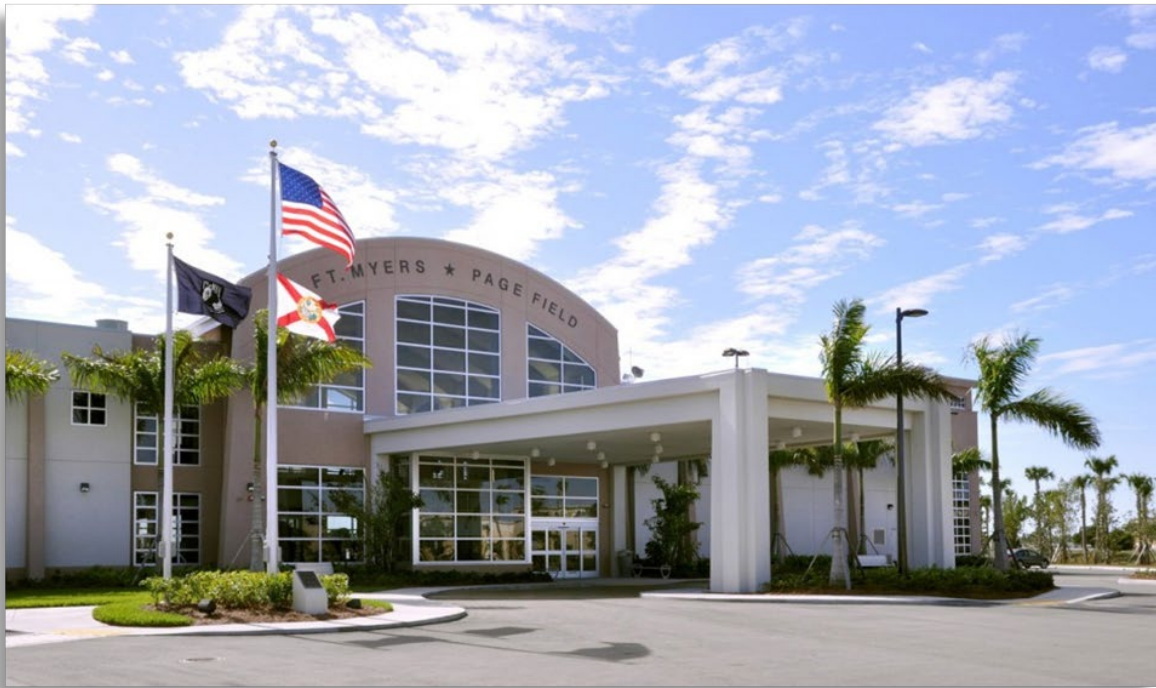
CONCRETE STUCCO EXTERIOR & ARCH'D ROOF & COVERED DROP OFF
