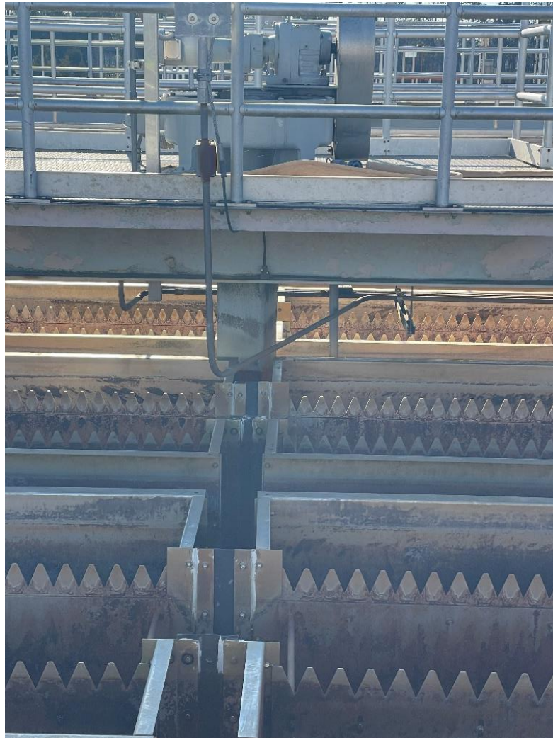
Photograph 2: Existing Drive Unit and Torque Tube
