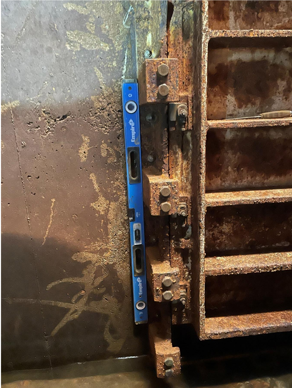
Photo 5: Existing Ozone Outlet Channel 2 Gate After Cleaning
