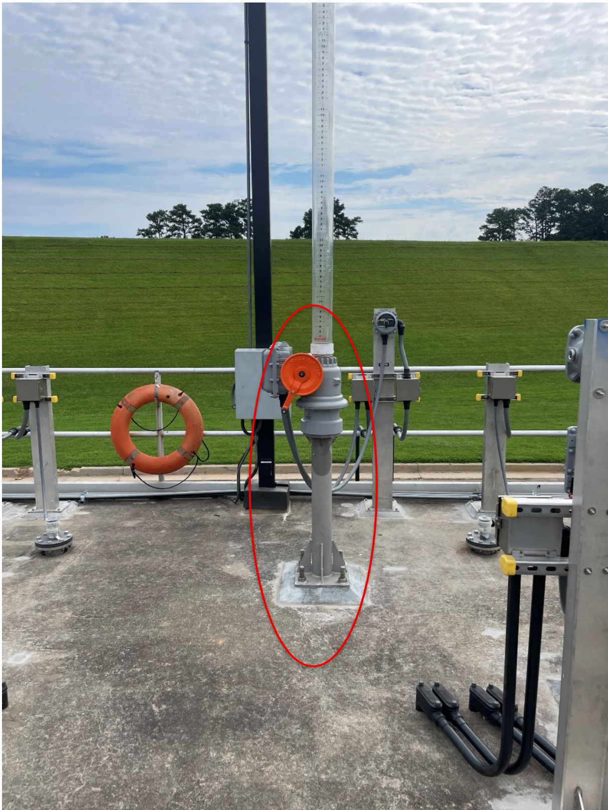
Photo 2: Intermediate Gate Operator
